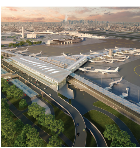
The detailed Tutor Perini/Parsons, JV, website ( www.tpcparsonsjv.com ) says that the Terminal One project also includes the N60 Frontage Road Bridge and pedestrian bridge with moving walkways. In addition, the scope of work involves site clearing, a
